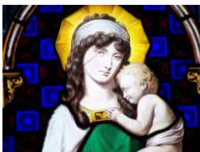
Caritas panel – window in S. Aisle(cracked)
